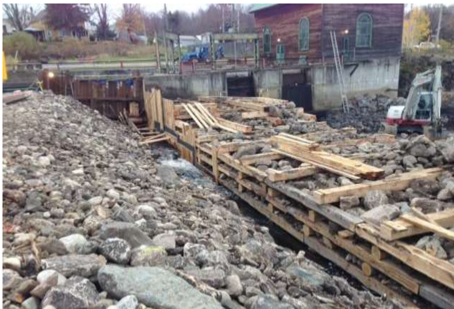
Figure 44: Lumber Crib dam under construction
